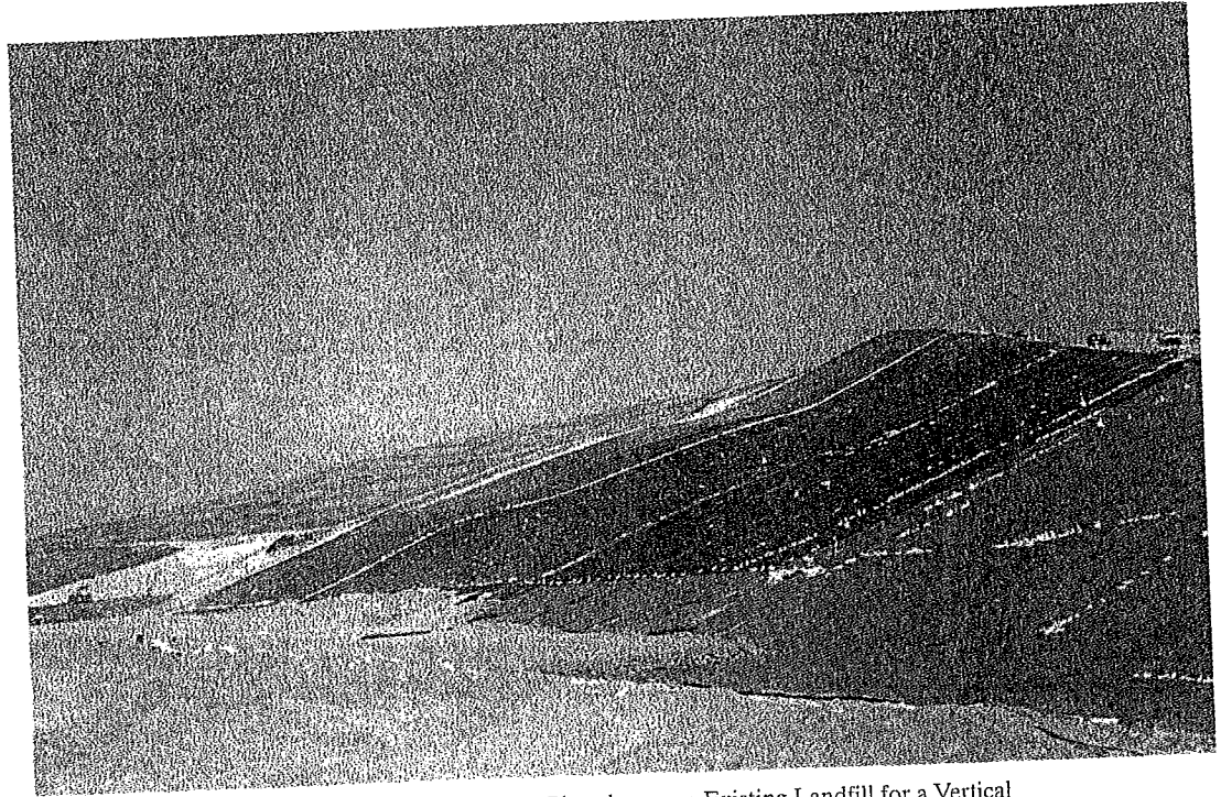
FIGURE 14.5 A Liner System Placed over an Existing Landfill for a Vertical Expansion Project
