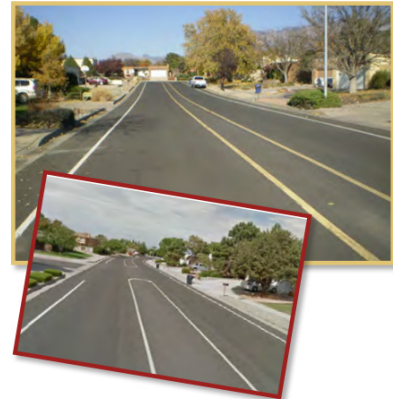
Figure 6: Centerline/Edge line/Lane Striping. Source: CABQ NTMP
