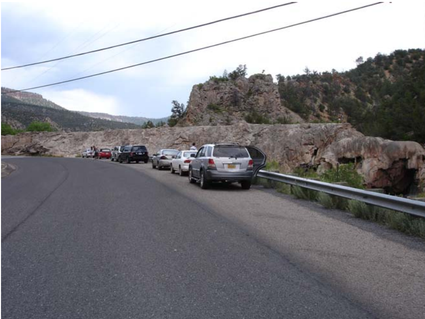
Unsafe Parking Conditions, Soda Dam
