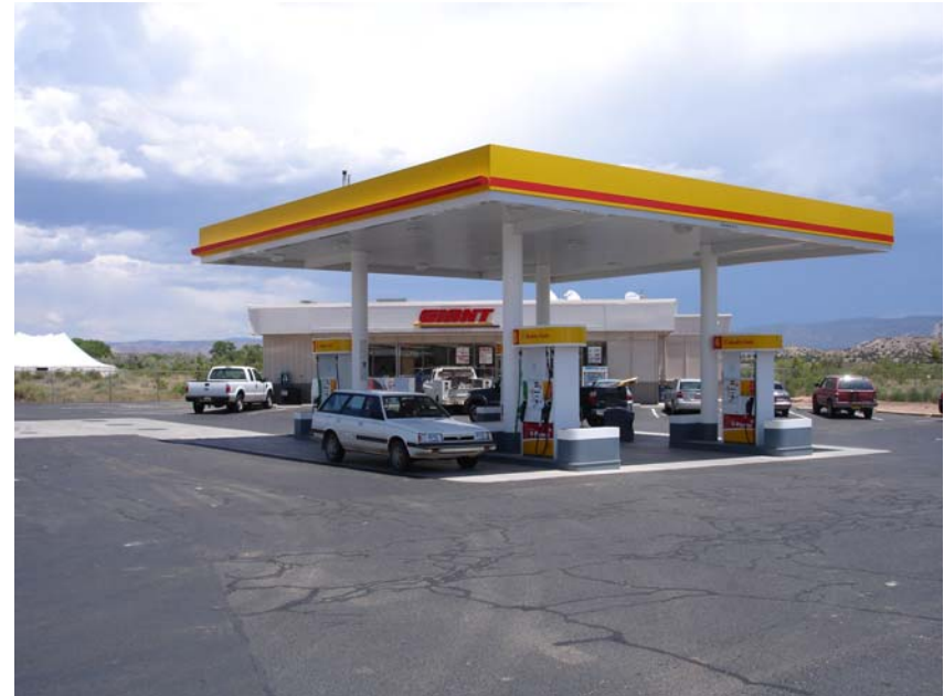
Commercial use on US 550 in San Ysidro
