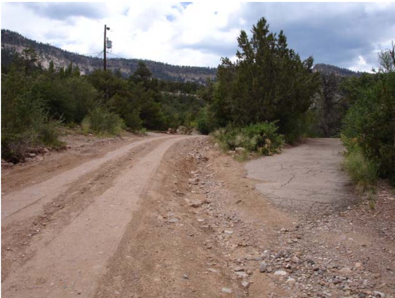
Road Runoff on Private Drive, Jemez Springs North
