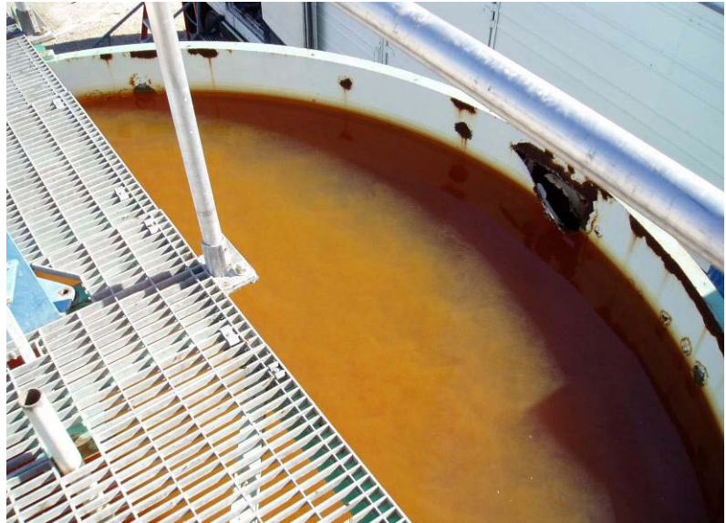
Clarification Using Ferric Chloride for Arsenic Removal 11/23/2009
