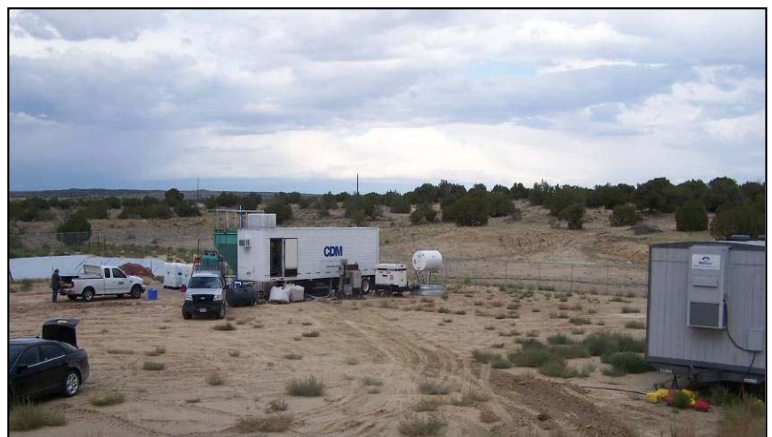
Sandoval County Desalination Pilot Facilities- September 2009
