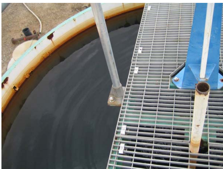
Figure 3-7 Unusual Black Water in Clarifier from Sulfur Oxidation
