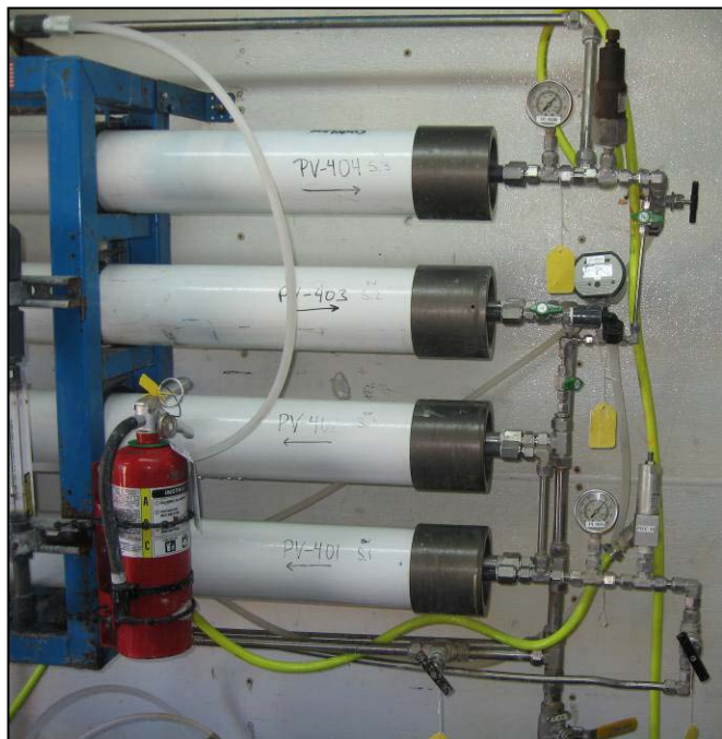
Reverse Osmosis Modules
