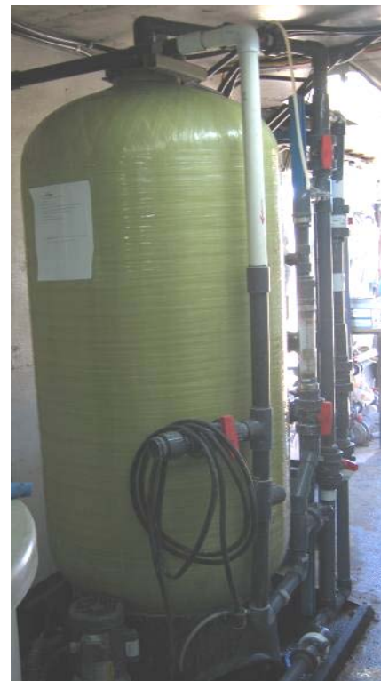
Figure 2-x Ion Exchange Pressure Vessels
